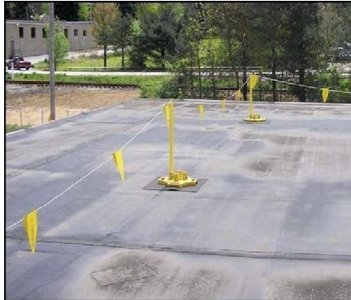
Warning Line System
