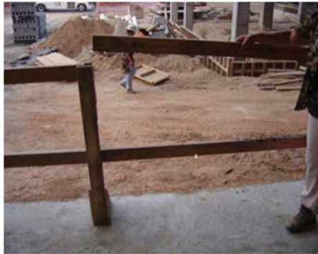
Removable Guardrail at second Floor
