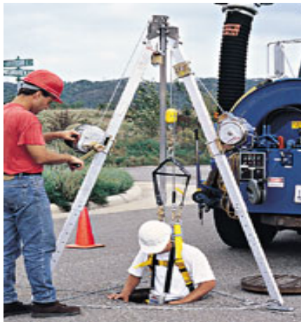
Tripod used for safe entry
