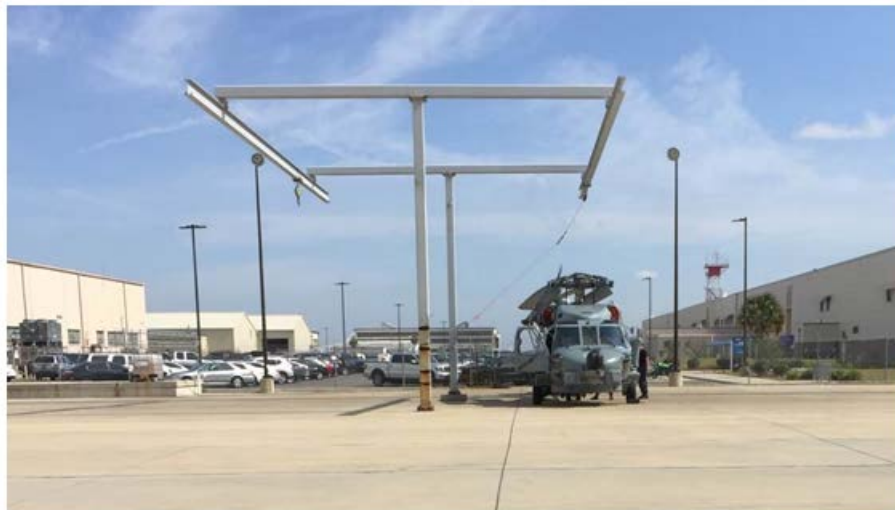
Figure 12. Wash rack facility.
