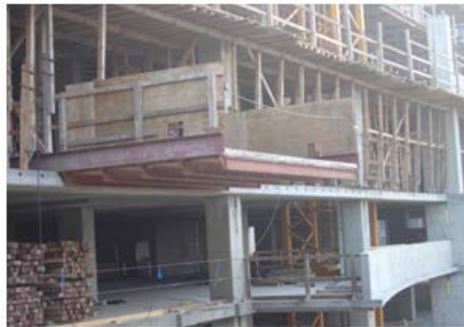
Loading Platform w/Removable Chain at point of access, however Mid Rail is also Required
