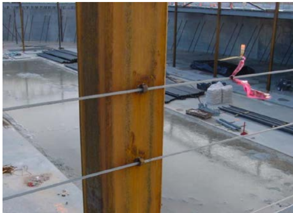
Steel Cable Guardrail
