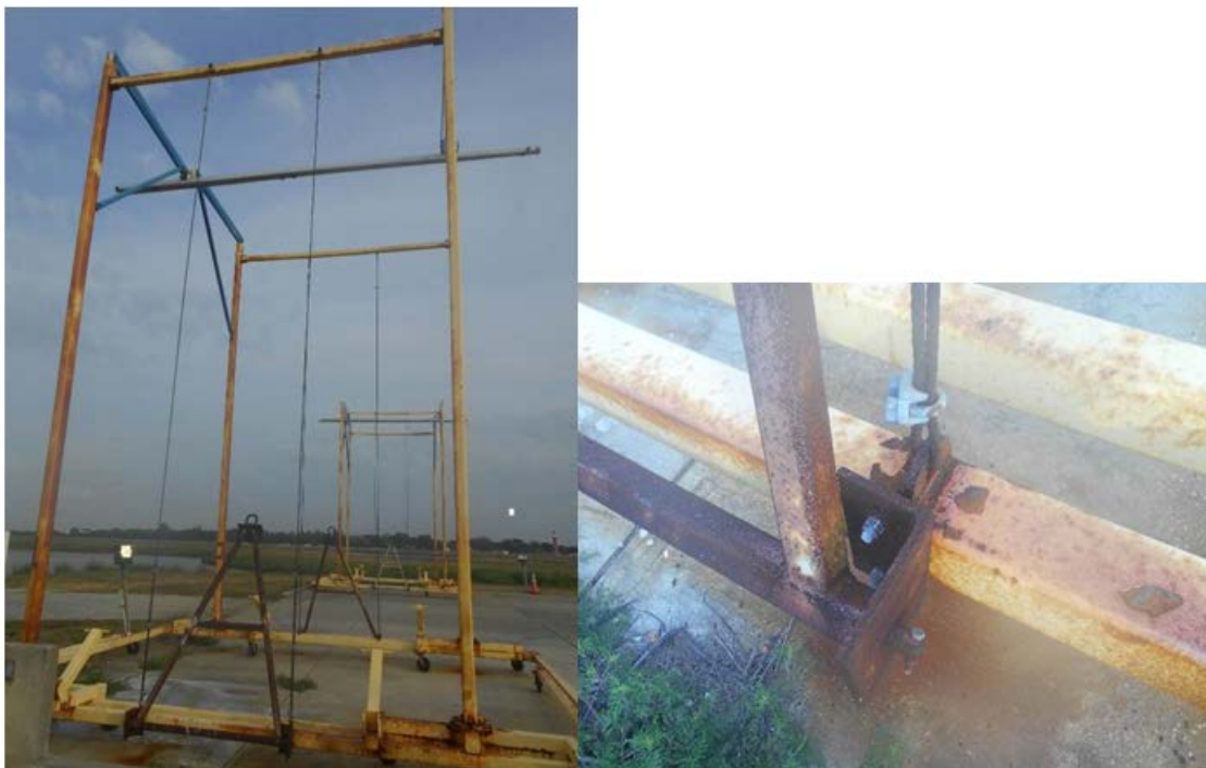
Figure 5. Corrosion issues noted on Webb-Rite Overhead Rigid Rail Systems located at the wash rack.
